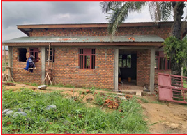
Photo 10 : Tshikapa skills Lab under construction
